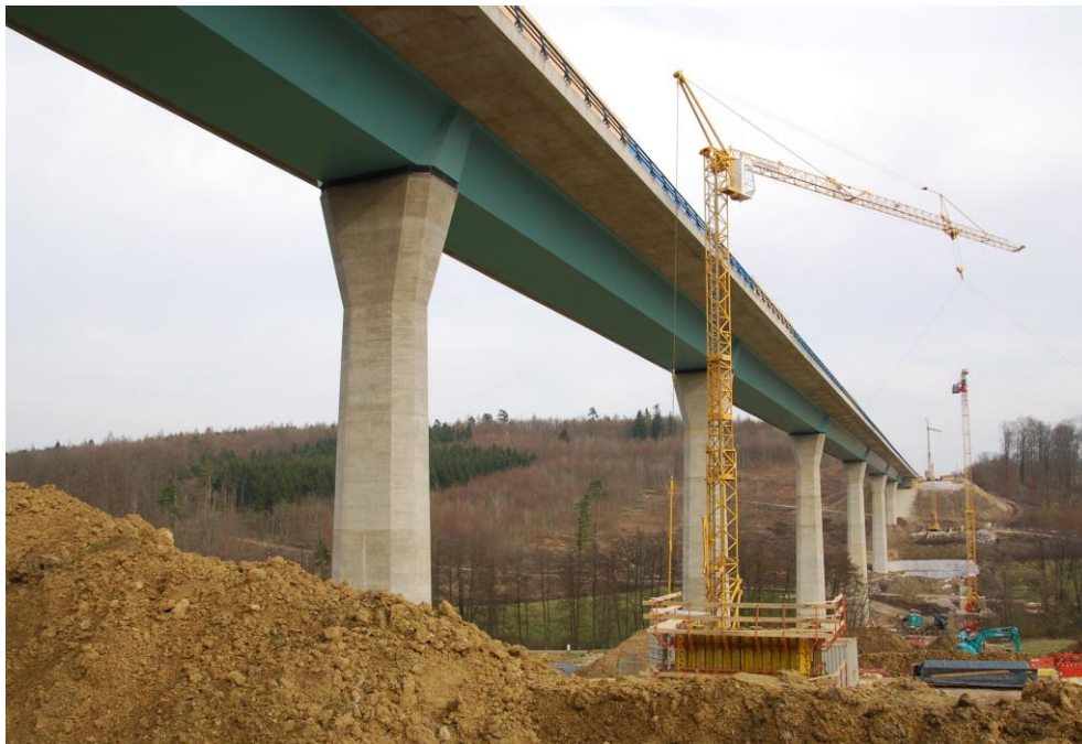
Figure 7. Dultenaugraben Bridge in Baden-Württemberg, Germany during construction. (CC 2008 Wladyslaw.)
