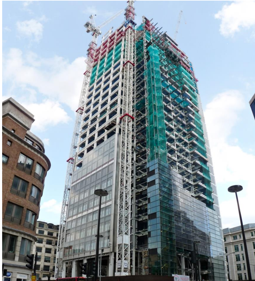
Figure 6. The Heron Tower in London under construction.
